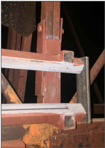
PHOTO 3 UPSTAGE PLATE LOWER TRACKS
